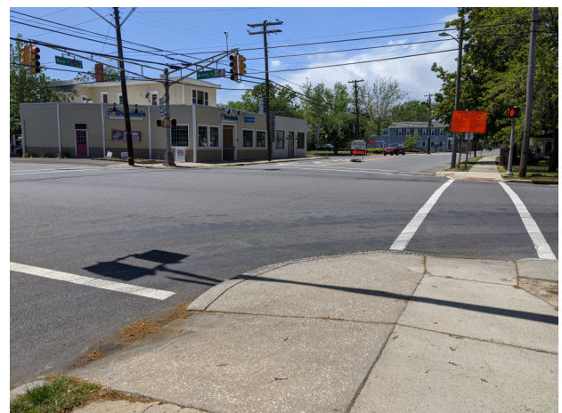
Non-ADA compliant curb ramps at the Main Street & Cape May Ave intersection
