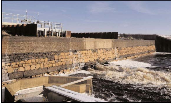
Lake Lenape Dam Photo Credit: Dave Griffin
