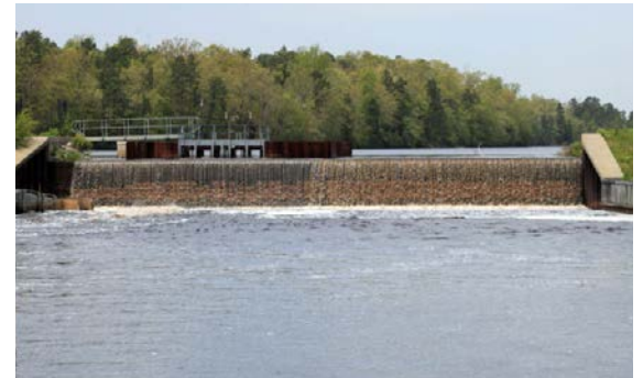
Lake Lenape Dam
